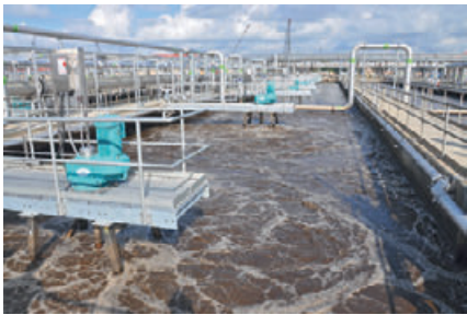
One of 90 Hyperclassic®-Mixer/Aerators in the Back River wastewater treatment plant in Baltimore, MD, USA (photo: HCMA)
