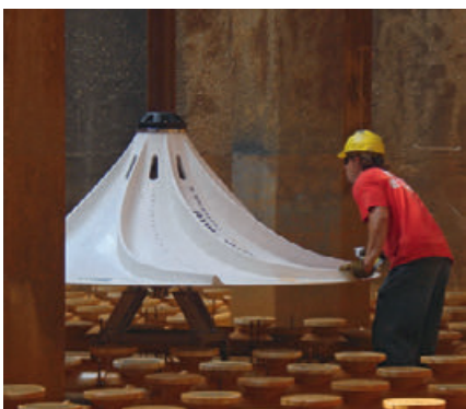
One of 112 Hyperclassic®-Mixers in the Blue Plains wastewater treatment plant in Washington, D. C., USA (photo: DC Wasa Photo)
