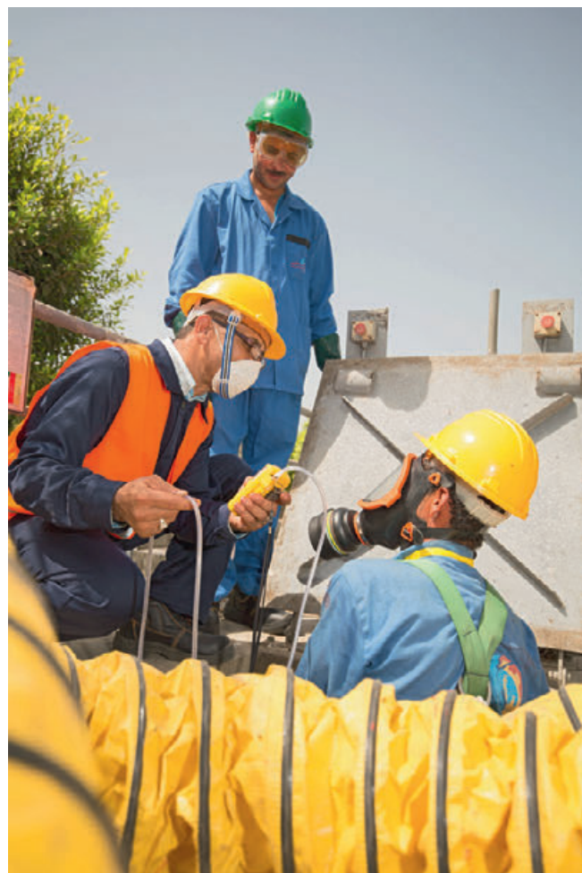
Safety first in a confined space
